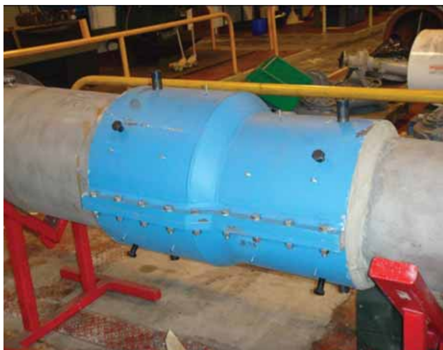
Figure 3: Repair of sleeve
