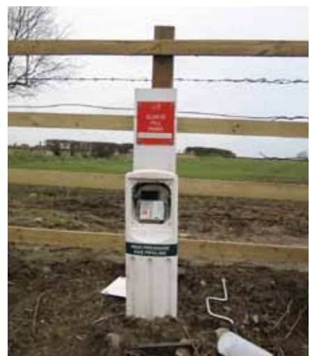
Figures 2A & 2B: Merlin nitrogen sleeve monitors
