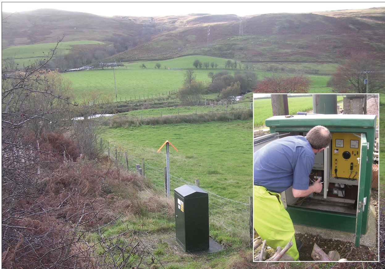
Fig.2. Many T/Rs are situated in remote locations where manual data collection (inset) is time-consuming.
