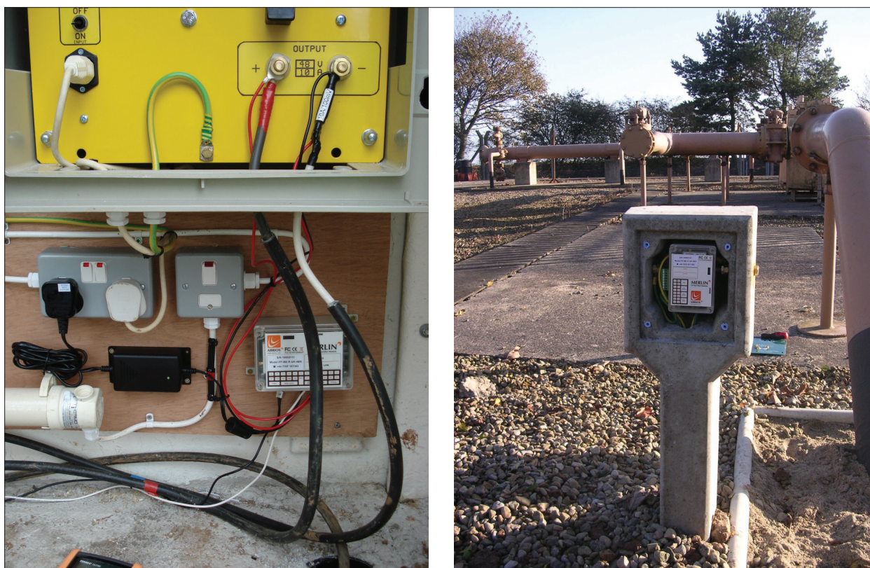
Fig.4. (a - left) Monitoring a T/R (Merlin unit lower right); (b - right) Monitoring a CP point at an above-ground installation.
