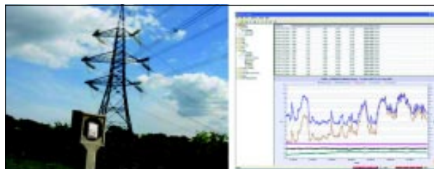
Figures 6a and 6b: Monitoring induced AC from power lines
