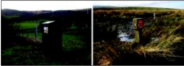
Figures 3a and 3b: Many CP T/Rs and test points are situated in remote locations where manual data collection is time-consuming
